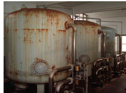
Condition of tanks before zinc tape application
