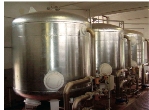
Condition of tanks after zinc tape application
